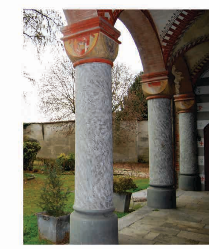
Stone columns have been painted.
