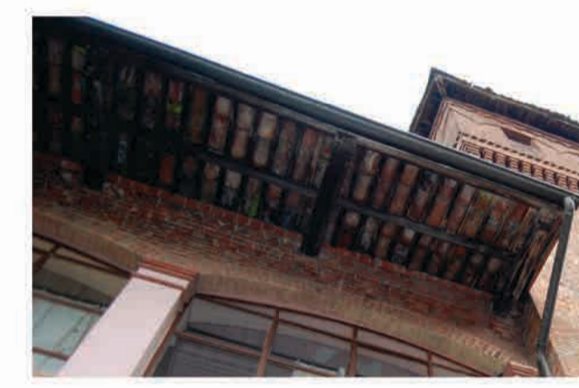
Wooden structure under roof
