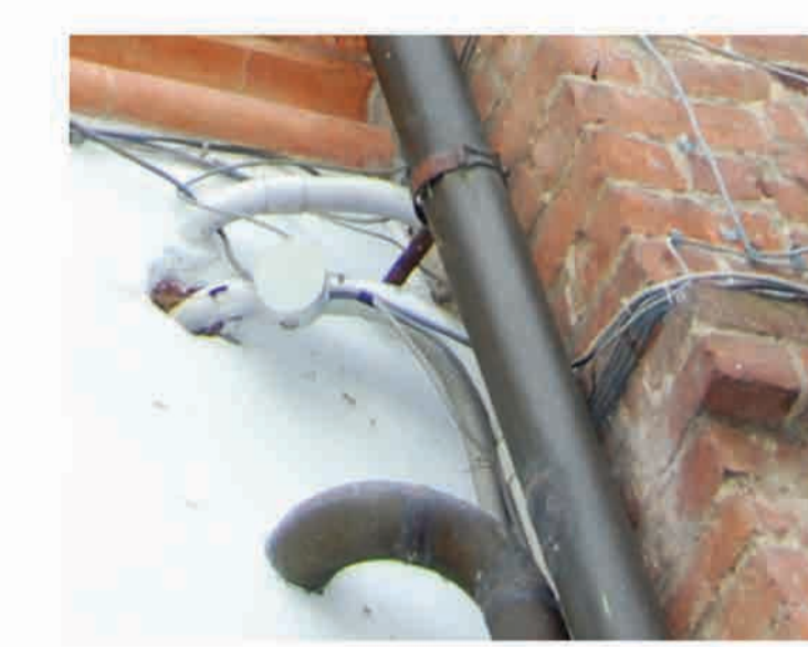
Plumbing feature and electrical connection holes on the facade.
