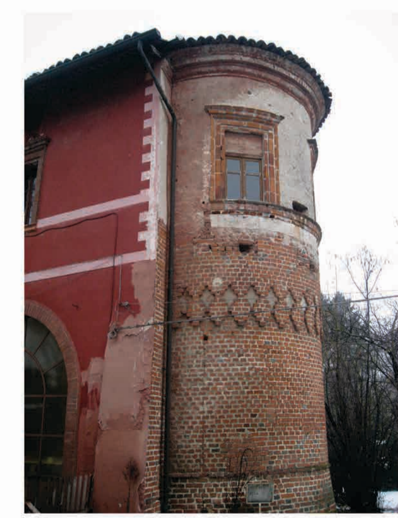
Plaster and brick exterior walls
