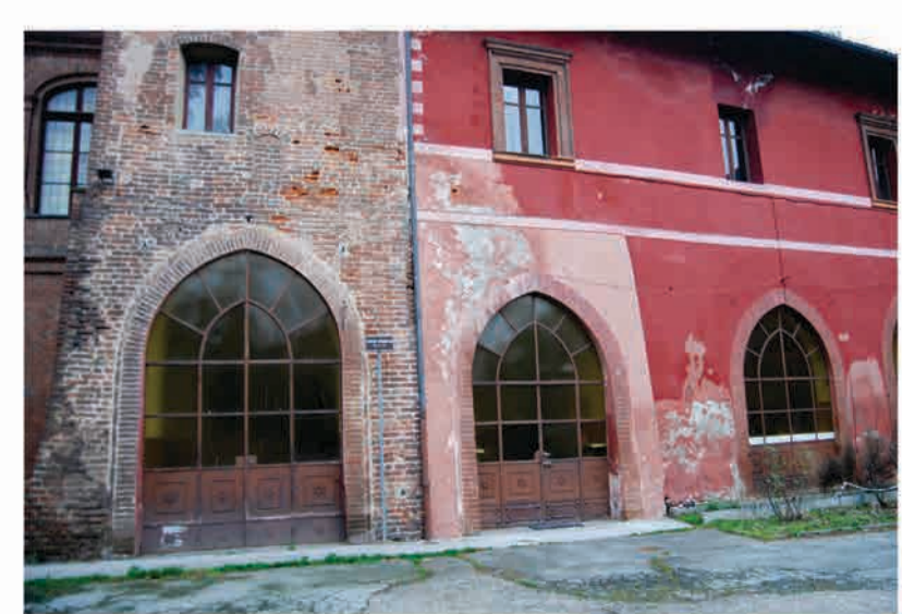
Plaster and brick exterior walls
