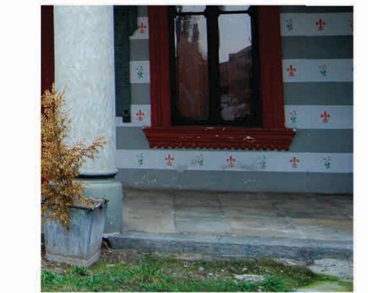
Floor on the entrance has stone and concrete.
